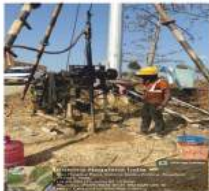
Drilling Rig for rock and Soil samples
